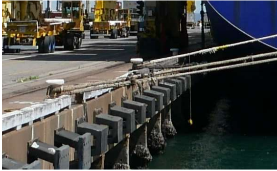
Figure 1 Fender System at Port Botany’s Brotherson Dock. The capacity of the closely spaced fender system is proportional to the hull radius at the point of contact.
